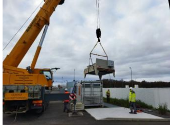
December 2024– beginning of 2025 Installation and Commissioning of HRS
