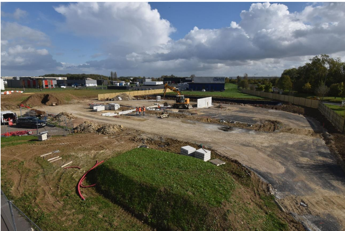
COSMHYC DEMO construction site, 24.10.2022. Picture © CCTVI
