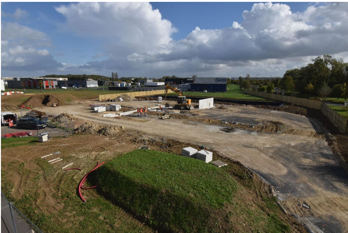
COSMHYC DEMO construction site, 24.10.2022. Picture © CCTVI
