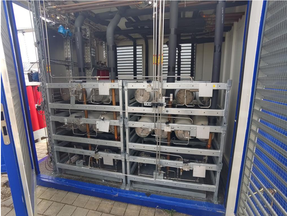
Metal hydride reactors in COSMHYC XL
