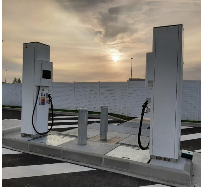
COSMHYC DEMO construction site, 12.01.2024. Picture © CCTVI
